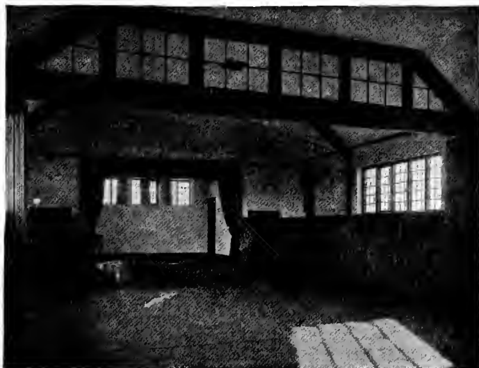
15.—INTERIOR OF HALL: SLIP END. P. Morley Horder.
